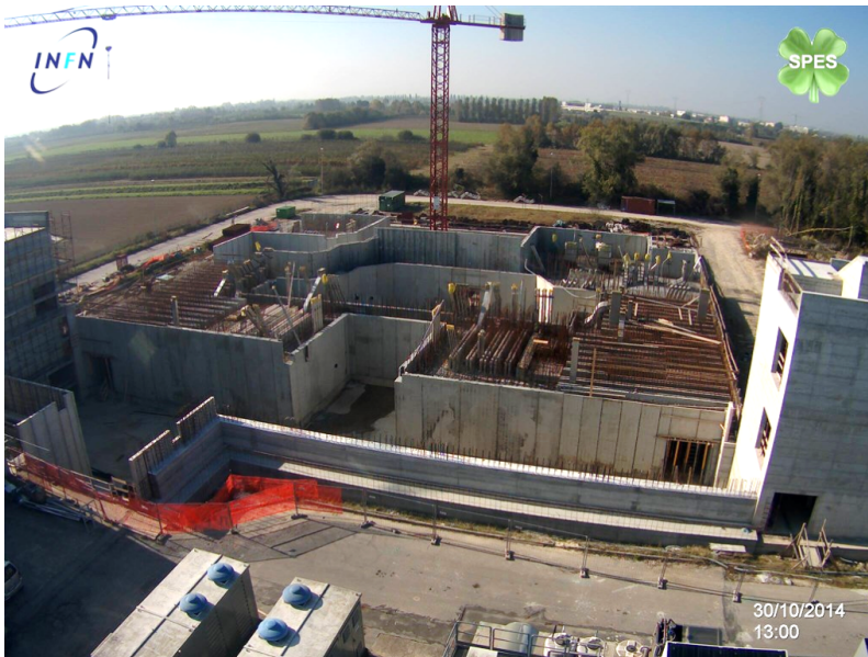
Fig. 7. SPES construction site.
