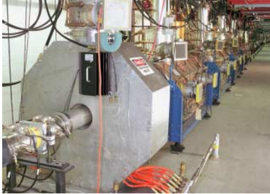
Figure 5.30. Finemet rf cavity with attached power amplifier
