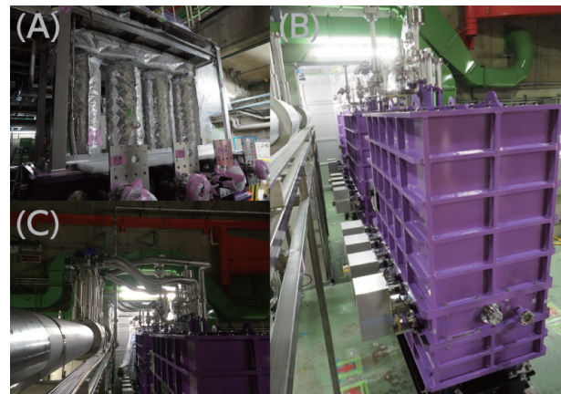
Figure 16: (A) Cryomodule in the final assembly, (B) Cryomodules after alignment, (C) U-tubes were connected between the cryomodule and the transfer line.
