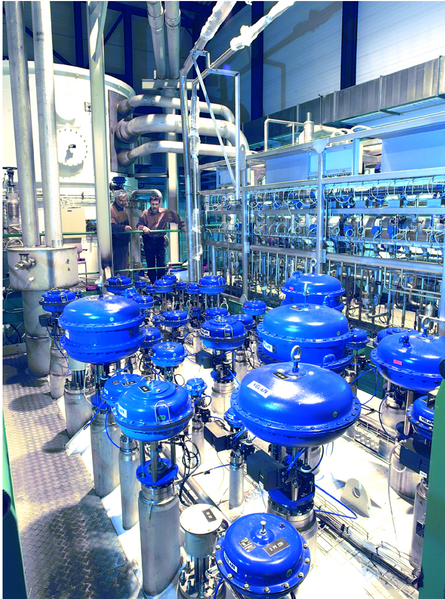
Figure 1.9: The cold boxes are major components of the LHC cryogenic system. This photo shows the top of the first cold boxes delivered to CERN
