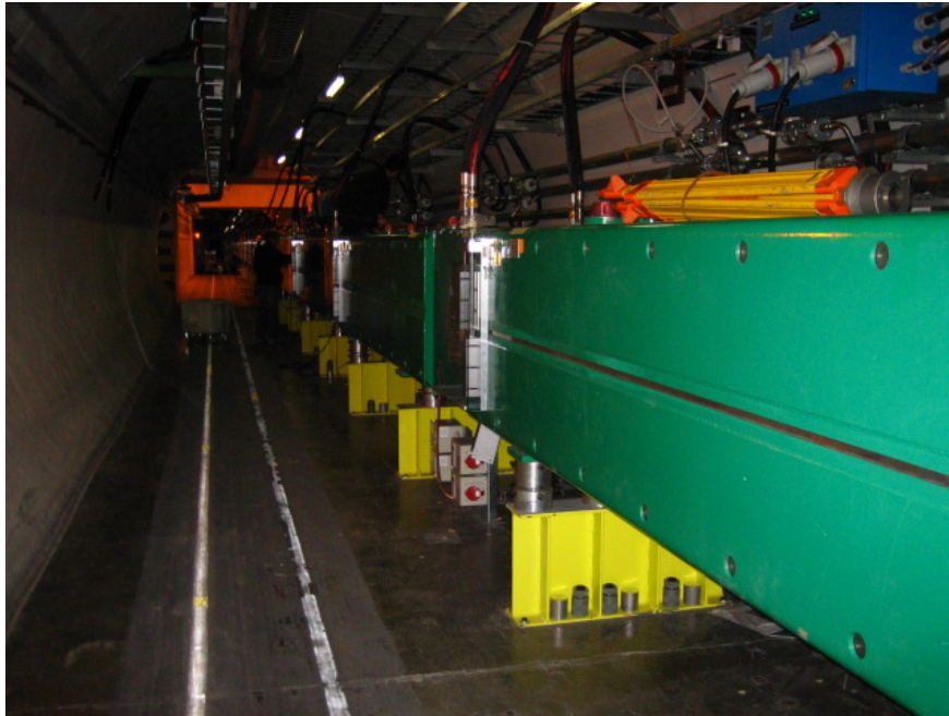
Figure 3.1: View of the MSD Magnets installed in the LHC tunnel
