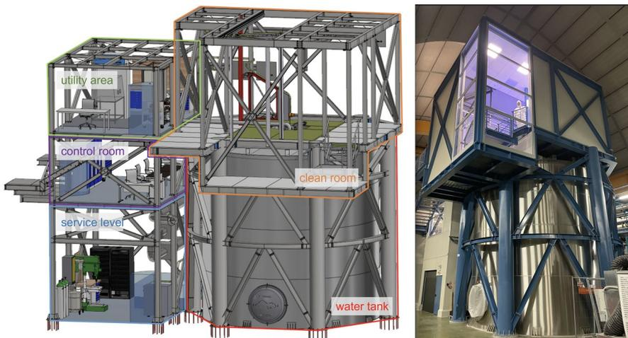
**Fig. 3** COSINUS facility located at LNGS. Left: Schematic view with control building and water tank. Right: On-site picture taken in August 2023
