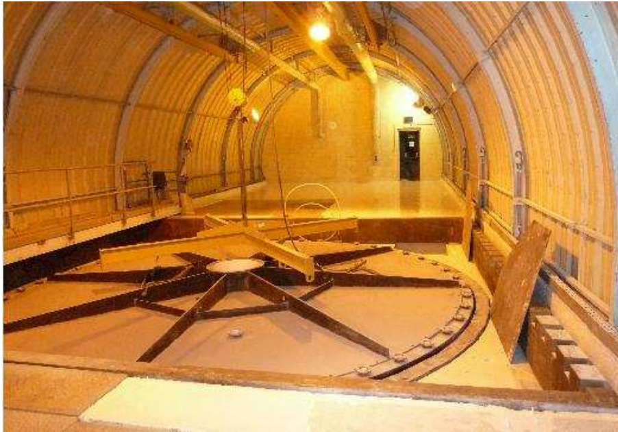
Figure 5. View of the far lab after the inner veto tank installation and ground painting. The cylindrical pit is covered in the picture with the inner veto lid.
