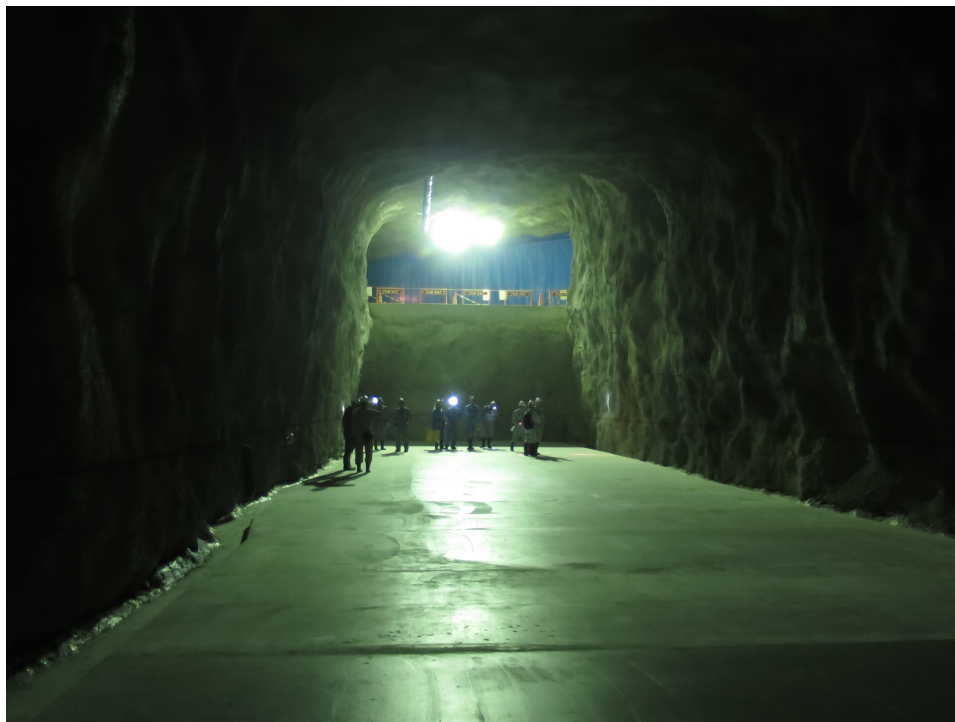
Figure 4. The newly-excavated Hall G. It will house the new water systems required to load Super-K with gadolinium and maintain its water transparency.
