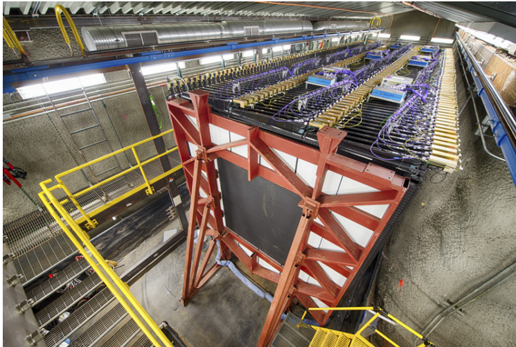
Figure 3.10: Photo of the Near Detector. The beam is incident onto the near edge of the detector. The top of the Near Detector shows the APD and FEB enclosures (gold colored boxes) wired to the central DCMs.
