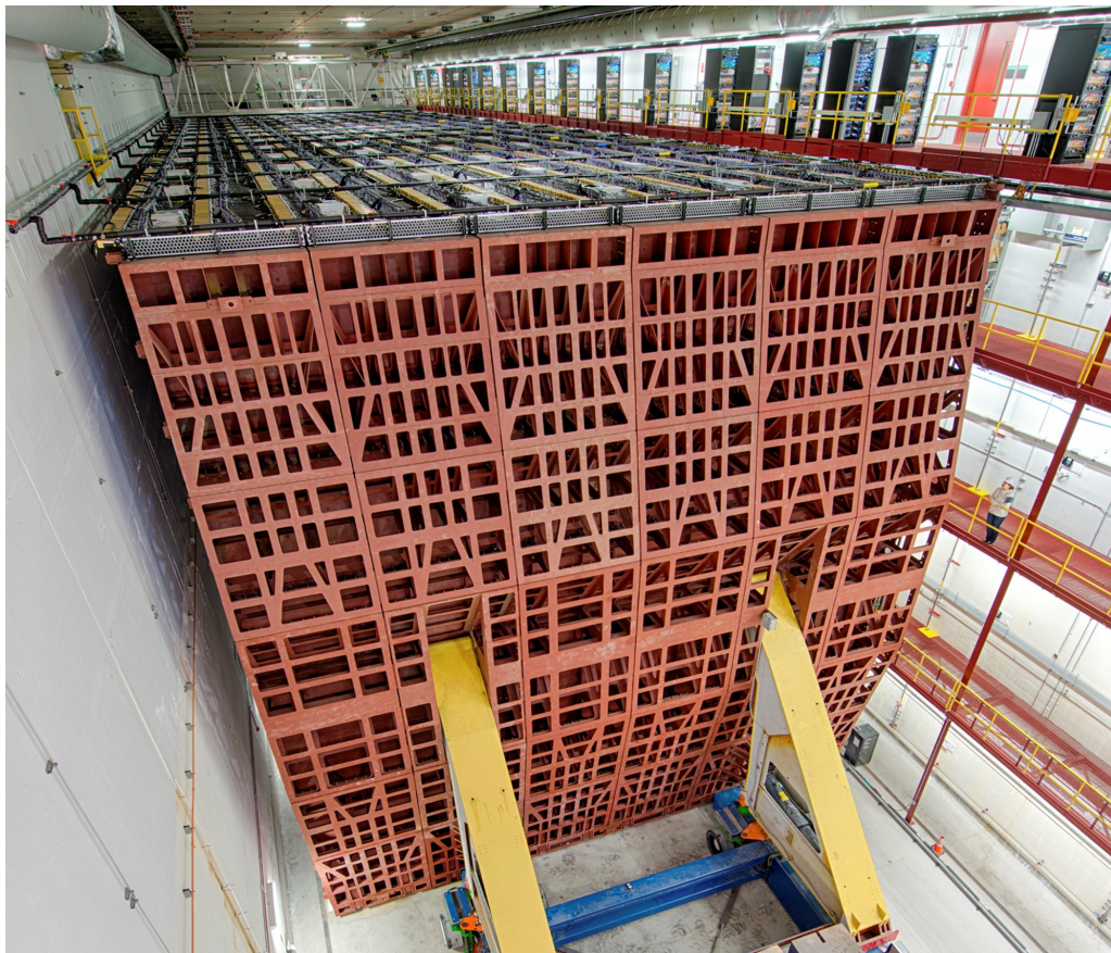
Figure 3.12: Photo of the Far Detector. The beam enters the detector from the opposite end than the one shown. The top of the detector is covered by the readout electronics (APDs, FEBs, and DCMs). The lattice of pipes above the electronics is the water cooling system that services the APDs.
