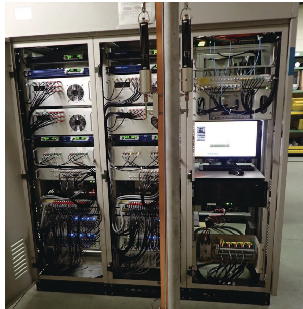
Figure 6: A photo of the standard unit for 4 quad and 4 steering magnets.
