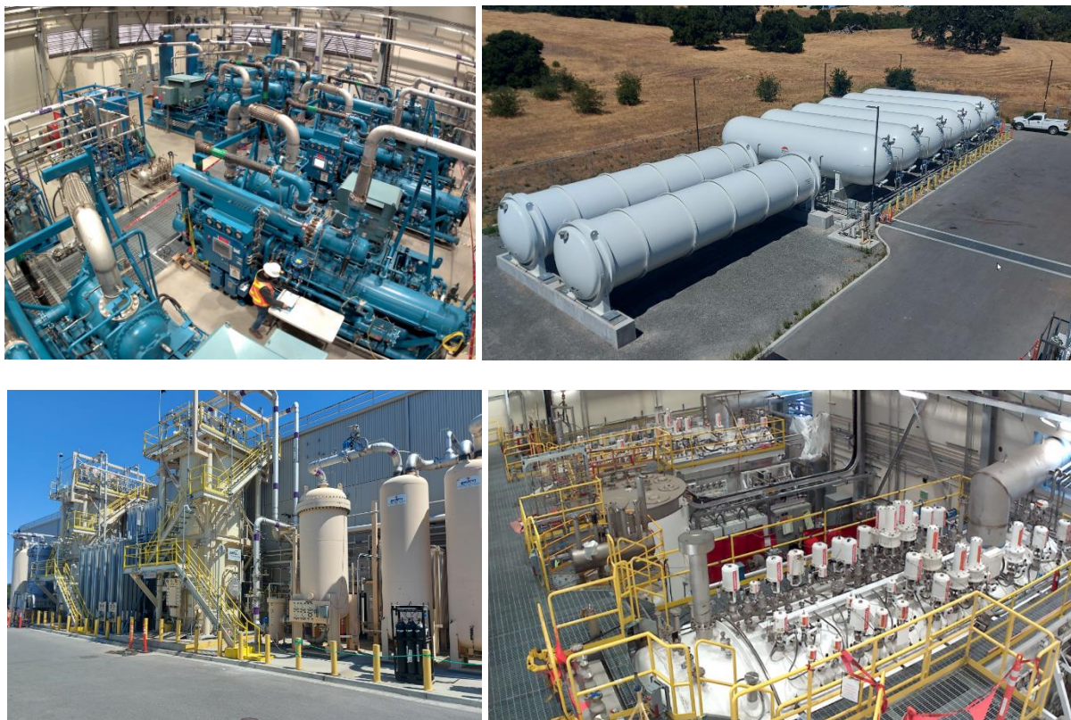
Figure 7. Upper left: Compressor room 1, Upper right: Tank farm with LN 2 and GHe storage tanks, Lower left: North slab installations with oil removal system, upper C1 and C2-CBX Lower right: Cold box room with lower C2-CBX, C2-10,000 I- LHD, C1-2 K CBX, C1-lower CBX
