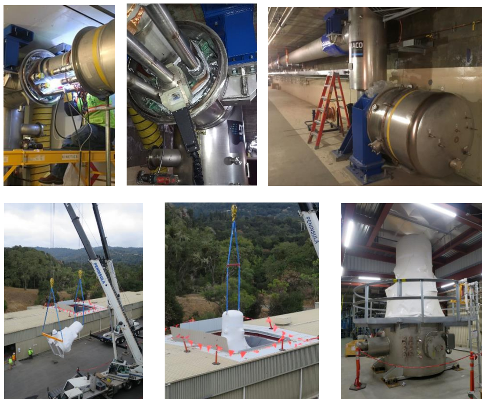
Figure 9. Installation of the tunnel transfer lines and distribution box installation in the klystron gallery through a roof opening.
