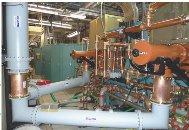
Figure 2: Coaxial feeders from PAs to branch hybrid.
