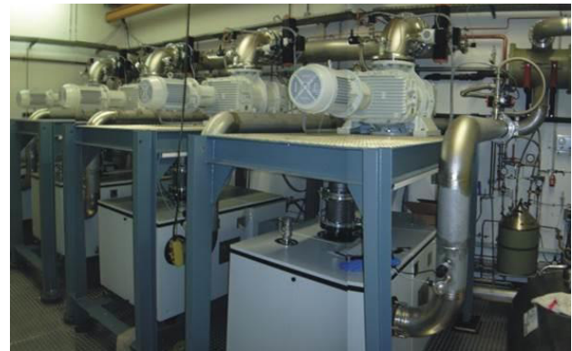
Figure 2: Four parallel switched Pumping Units.
