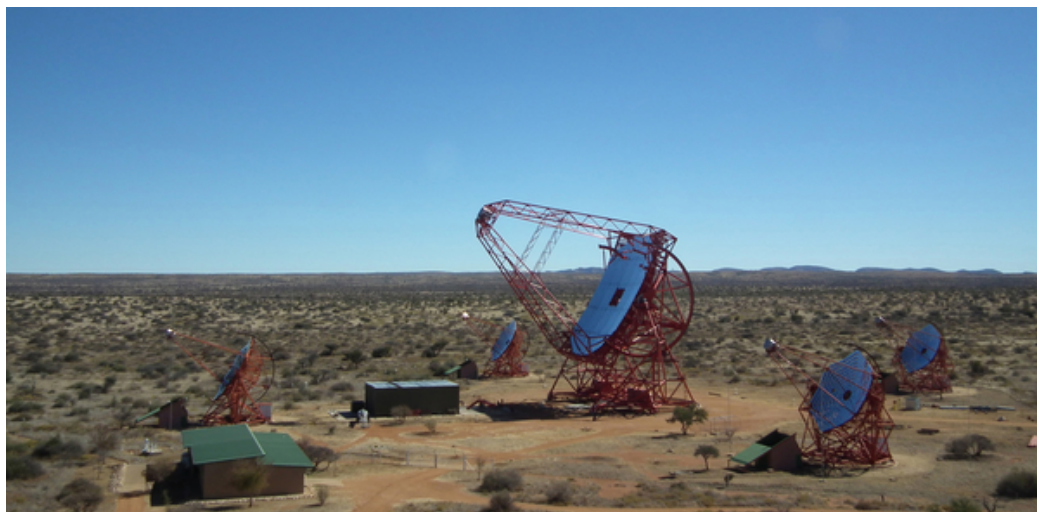
Figure 1.33: H.E.S.S. gamma-ray observatory in Namibia. The final array consists of four 12 m diameter telescopes arranged on a square of side 120 m and a parabolic 28 m diameter telescope located at the centre. H.E.S.S. is the only operating hybrid IACT array and its energy range covers from 30 GeV to 100 TeV. Image credit: H.E.S.S. Collaboration; https://www.mpi-hd.mpg.de/hfm/HESS/pages/about/telescopes/ , last accessed on 01/08/22.
