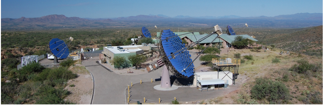
Figure 1.32: View of the FLWO basecamp and the 4 telescope VERITAS array at the base of Mount Hopkins in southern Arizona, USA. Designed to detect gamma-rays in an approximately energy range of 50 GeV to 30 TeV, the full array configuration started operations in September 2007 and it was upgraded in 2009. Image credit: VERITAS Collaboration; https://veritas.sao.arizona.edu/ , last accessed on 01/08/22.
