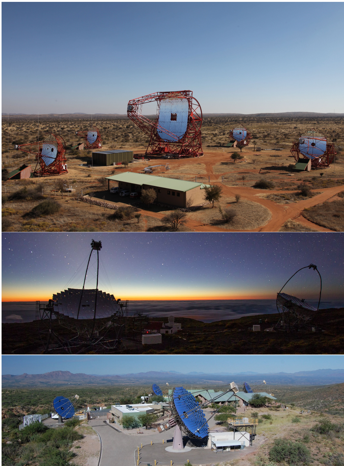
FIGURE 1.11: From top to bottom: the HESS (4+1) array of IACTs located in Namibia, consisting of four 12 m diameter and one 28 m diameter telescopes; the two 17m-diameter-dish array of MAGIC located on the Canary Island of La Palma; the four 12 m diameter IACT array of VERITAS located at Mt Hopkins, Arizona.
