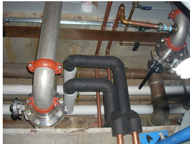
Figure 5: New Chilled Water Lines (insulated pipes in this photo).
