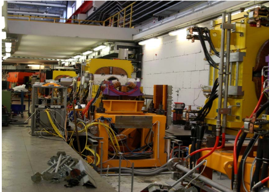
Figure 7: Preparatory work for the installation of low- \beta quadrupoles at the PAX target point in COSY, as of July 2009
