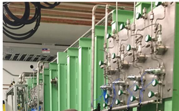
Figure 16: Pneumatic tuner manifold for the  $\beta = 0.53$  HWR cryomodule.
