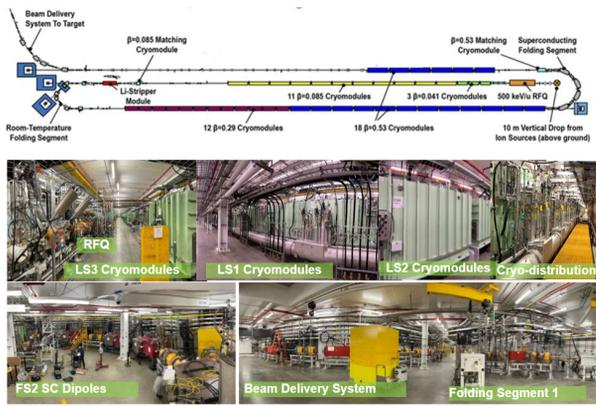
Figure 3: Layout of the driver linac, with photographs of equipment in each linac segment (LS1, 2, 3) and folding segment (FS1, 2).
