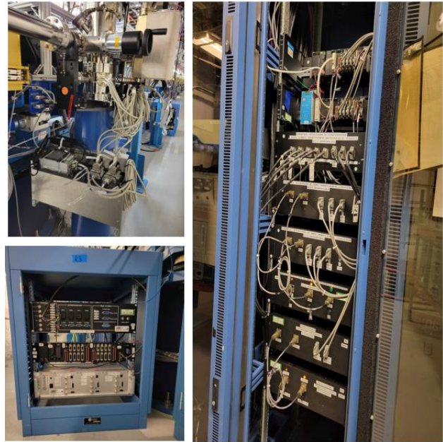
Figure 10: Clockwise from top left: station C fixture to hold the motor controller, station E and F motion control rack, and one of the C1 motion control racks.
