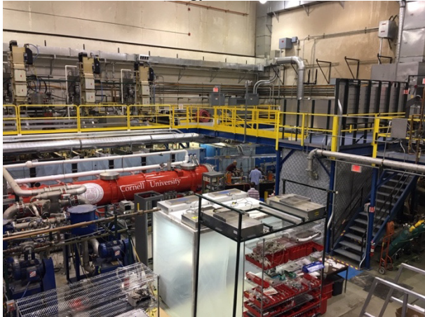
Figure 2: The superconducting six module linac MLC the major part of CBETA project.
