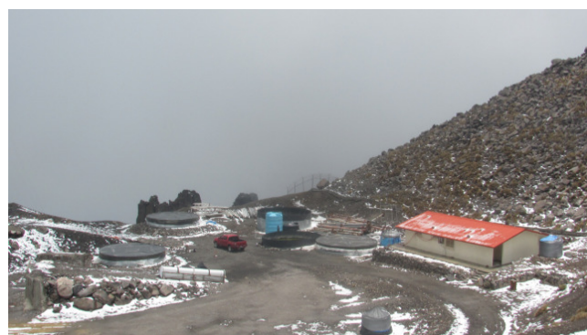
Figure 4: LAGO Sierra Negra WCDs. The old array of small tanks are clearly seen between the new big stainless steel tanks. Those are covered by an black EPDM liner.
