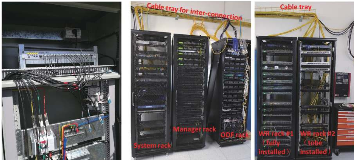
Fig. 56. (color online) WRS installation in 1#PDR.
