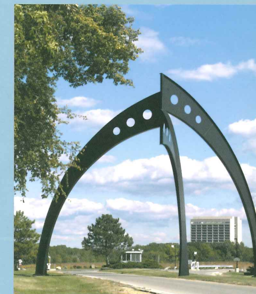
Broken Symmetry towers 50 feet above the Lab's west entrance. Robert Wilson designed the 212-ton structure, which was built in the Lab's machine shop. Some of the steel came from the decommissioned USS Princeton .
