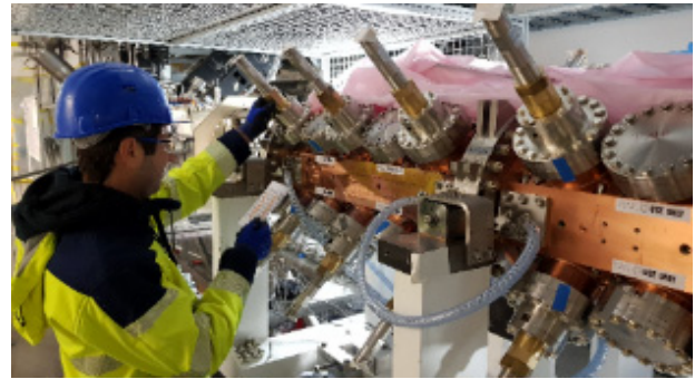
Figure 5: tuner position adjustment.
