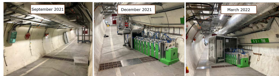
Figure 3. Detector installation in the TI18 tunnel.
