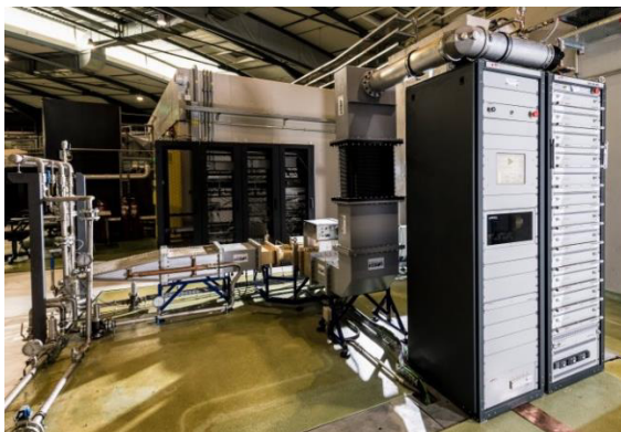
Figure 5: SSPA transmitter for the ALBA booster.
