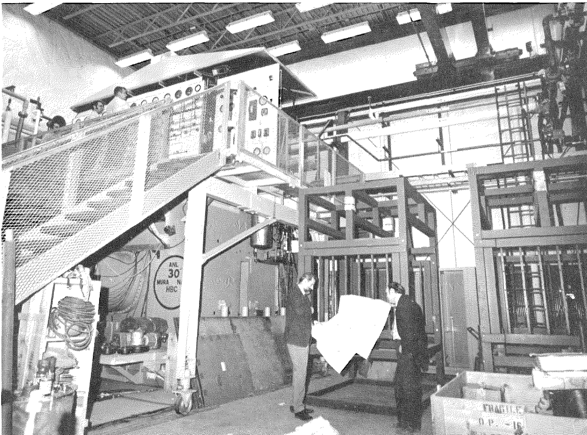
Fig. 1. While the bubble chamber is being readied for cooldown, components of the downstream wide-gap spark-chamber equipment are beginning to be installed. Lou Voyvodic and Ron Walker are looking over the spark-chamber plans while Dick Brazzale, Gary Hodge, and Del Wilslef are working on the upper platform.
