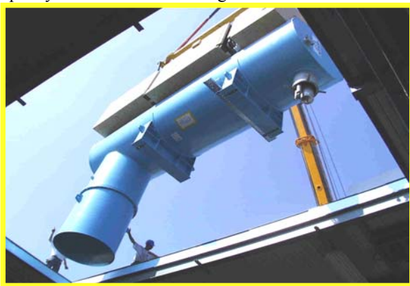
Figure 3: IHI/Linde 1.8 K cold box.
