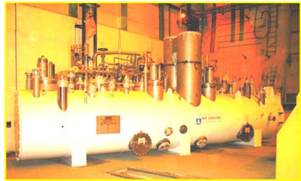
Figure 2: Cold box of the QUI at point 8.
