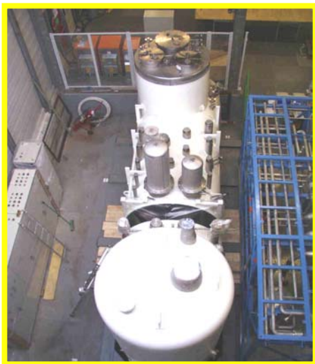
Figure 4: Air Liquide 1.8 K cold box.
