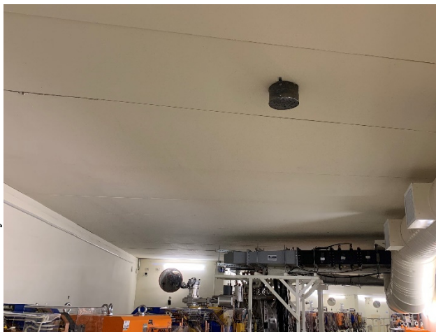
Figure 6: Smoke detector with lead shielding.
