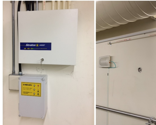
Figure 7: Aspirating smoke detector installed in the CIA room outside of the tunnel (left) and sampling pipes in the tunnel (right).
