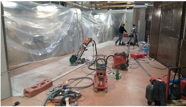
Figure 7: Levelling activities on the EH floor.
