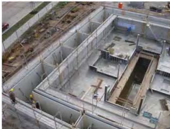
Figure 14: Basement for a huge bunker for a linac-based material testing site, which will be completed with a linac CT
