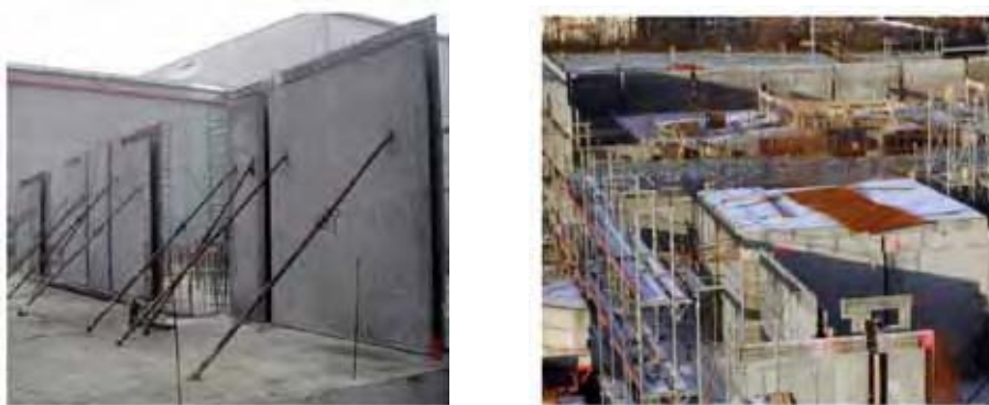
Figure 14: Basement for a huge bunker for a linac-based material testing site, which will be completed with a linac CT
