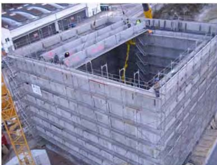
Figure 16: Closing the house top with pre-cast concrete girders, which will also be filled with mineral aggregate
