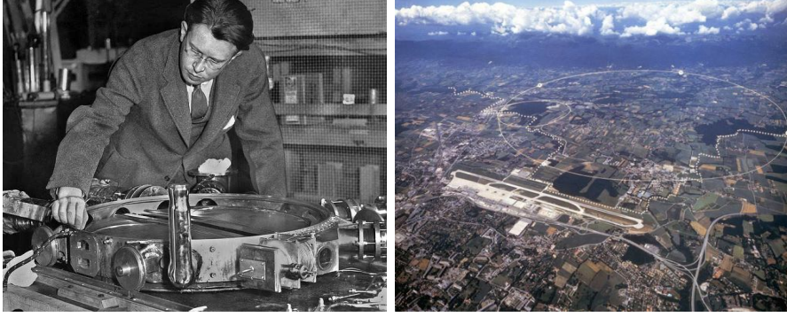
Figure 2.1: Lawrence’s cyclotron [Courtesy of University of California, Berkeley] (left), aerial view of LHC [Courtesy of Lawrence Livermore National Laboratory] (right). The dotted line depicts the Franco-Swiss borders while the full white circles represent the interaction points where the four major LHC experiments are installed.
