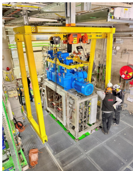
Figure 4: ATLAS underground installation.
