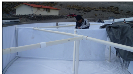
(a) Installation of Tyvek walls inside a tank.
