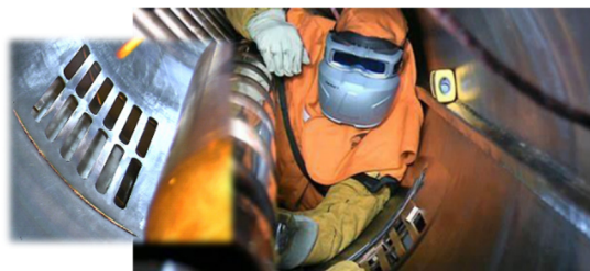
Figure 3: LANSCE DTL repair. Crack shown in left image. Welding repair in in right image.
