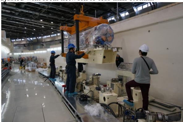
Figure 10: Girder installing with a cradle by a crane
