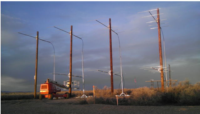
Figure 7: Fixed azimuth phased Yagi-Uda radar transmitter array. Wood masts allow vertical or horizontal polarization. Maximum power handling is 40 kW, equivalent to over 8 MW effective radiated power.
