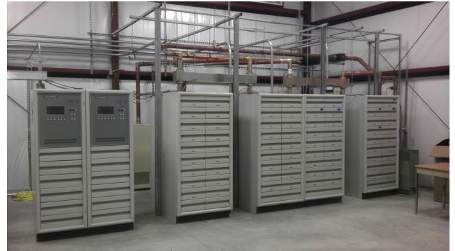
Figure 5: TARA40 radar transmitter is comprised of two 20 kW analog TV transmitters. Modifications have been made to broadcast a single 54.1 MHz tone with 100% duty cycle.
