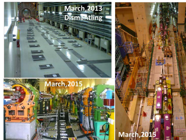
Figure 4: The beam line of ~320 m around IR has been reconstructed completely.
