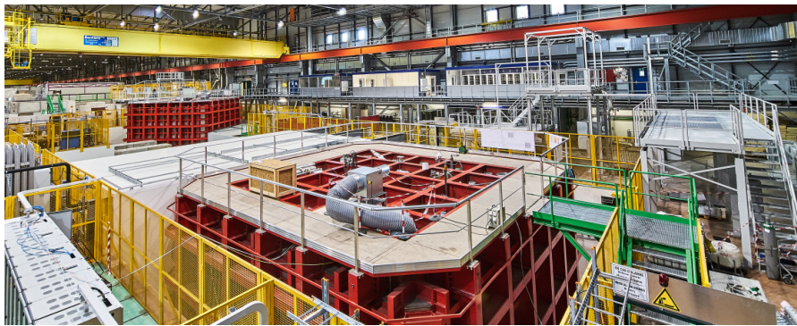
Figure 7. ProtoDUNE-SP and ProtoDUNE-DP cryostats in the CERN Neutrino Platform
