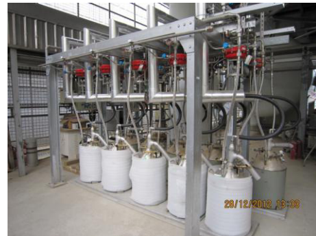
Figure 3: Two arrays of purifiers cooled with liquid nitrogen.
