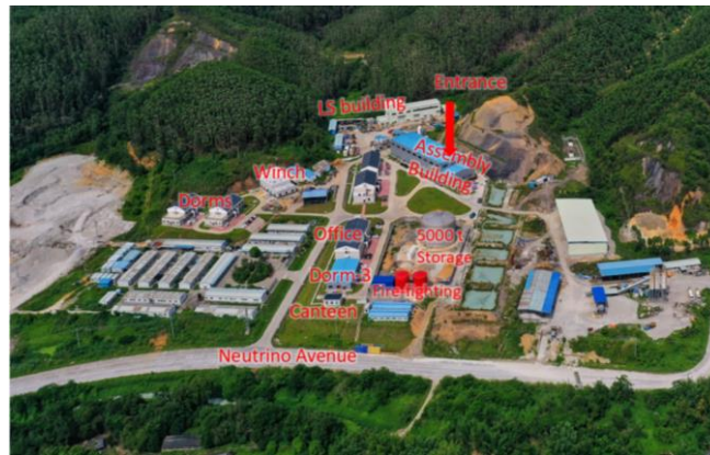
Fig 5: The latest (July) status of JUNO onsite surface building
