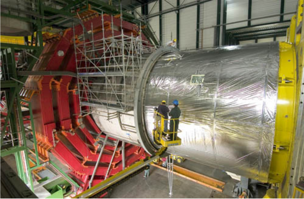
Figure 3.8: The CMS magnet during construction. The cylindrical magnet coil and the return yoke (12-sided red structures) are shown (this figure is taken from [90]).
