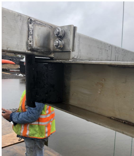
Figure 4.8: A mounting bracket welded to the main frame to which a stringer was bolted.
