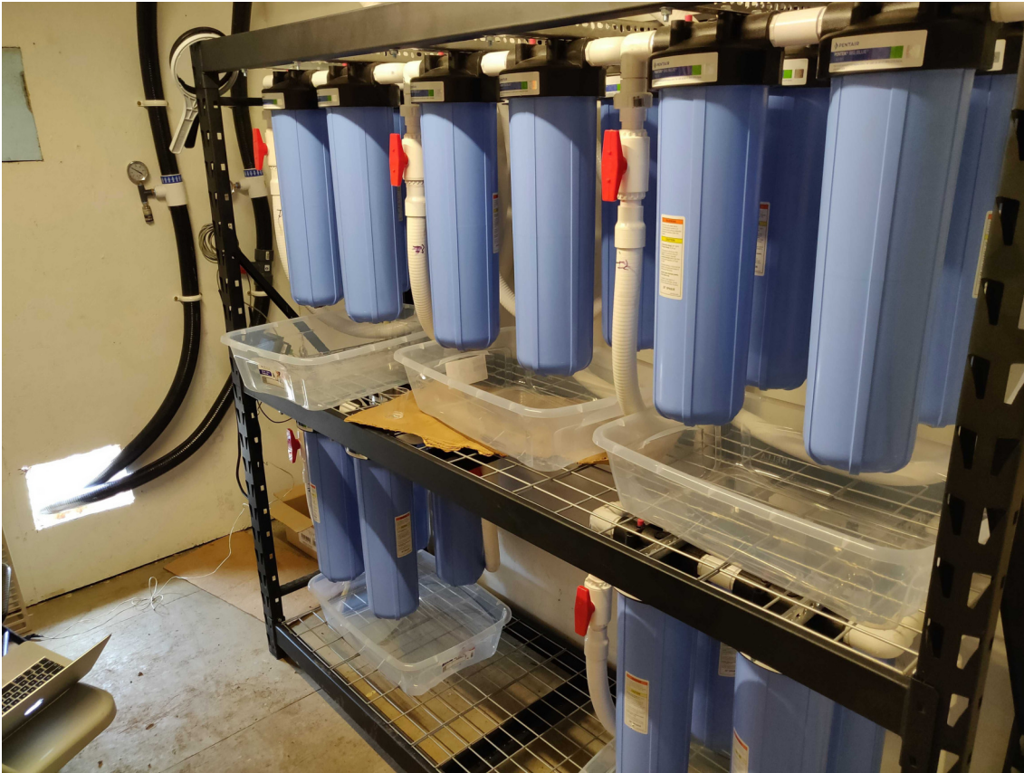
Figure 4.16: The interior of the water hut showing the filters. Image courtesy of Thomas Dodwell.
