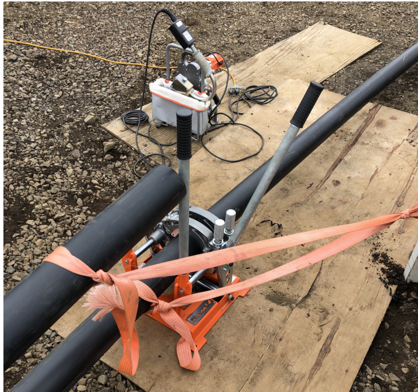
Figure 4.18: The equipment used to butt weld two sections of HDPE pipe together. The ends of the two pipes were shaved down to be smooth and flush with each other. A heated plate was placed in between until the ends had melted. The two sections of pipes were pressed together and the melted sections were fused together. The process was precisely controlled for standardised joints.
