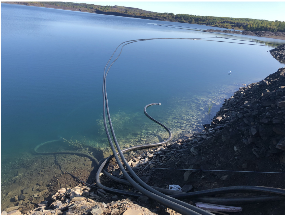
Figure 4.19: The completed inflow and outflow water pipes for the detector. The short pipe on the surface is the water intake for filling the detector during deployment.
