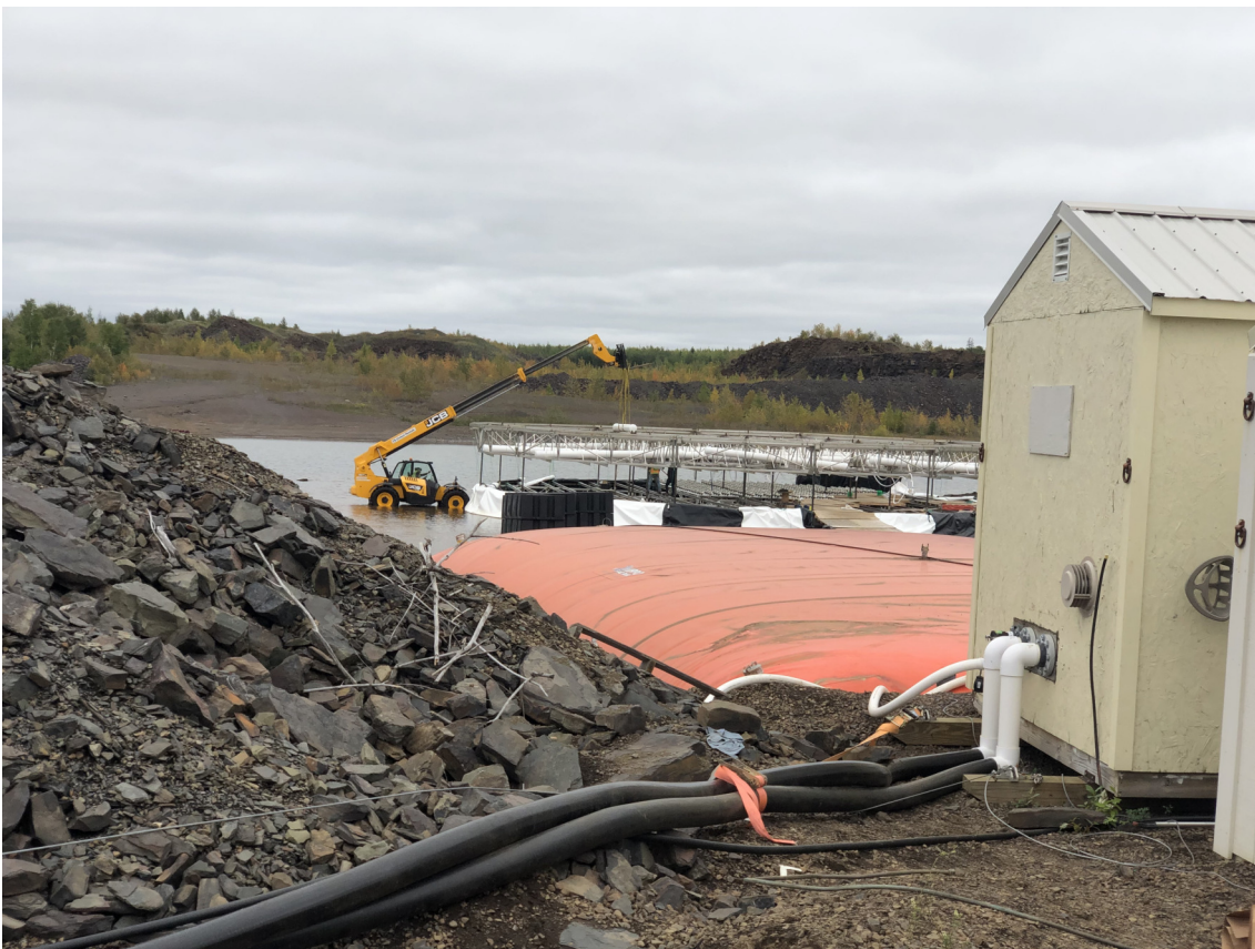
Figure 4.17: The exterior of the water hut showing the passthrough between the black HDPE pipe and the inside of the hut.
