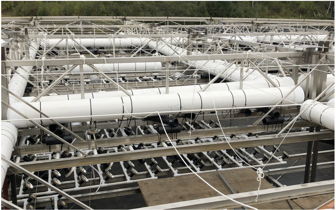
Figure 4.12: The 12 inch PVC buoyancy pipes mounted in the top cap to provide flotation.
