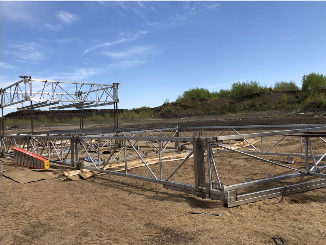
Figure 4.6: Pieces of the bottom end cap. The gusset plates used to join pieces are visible as are the tyres which the frame sits on. The hollow lattice style design saves weight as less steel is required than for a solid detector.
