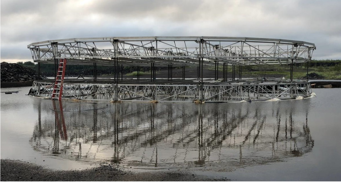
Figure 4.9: The completed frame. The pillars supporting the top cap are clearly visible.
