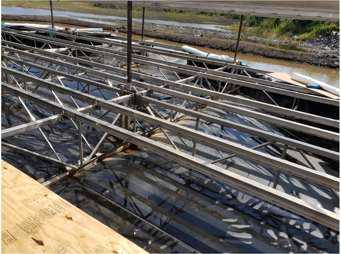
Figure 4.7: Rows of stringers bolted to the main support structure. Detector planes would be attached on top of the stringers.
