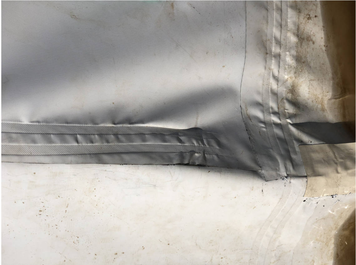
Figure 4.10: Two pieces of liner fused together (unfinished). Hot air is blown in the gap between the two pieces until the melting point is reached. The two pieces of liner are clamped together. The joints were not individually tested due to the circumstances of construction. However, prior testing showed they were expected to be light-tight if properly performed.
