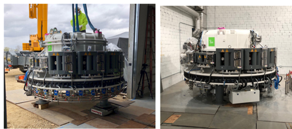
Figure 4: The first accelerator during (left) and after (right) rigging into its vault.
